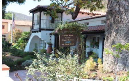
Water District Building
